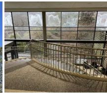
CVG Curtain Wall Window Project (State Funded)
